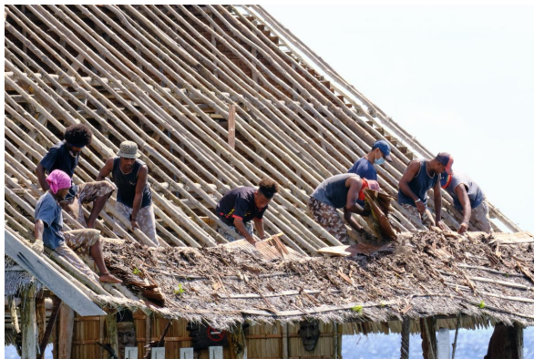
Taking off the old roof
